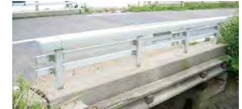
20years after the construction, with CFCC® reinforcements.
