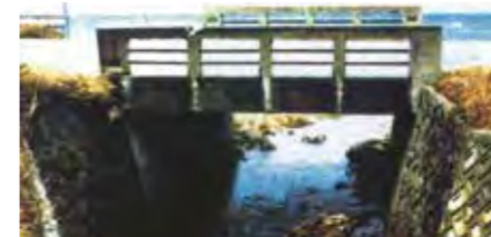
20years after the construction, with Steel reinforcements.
