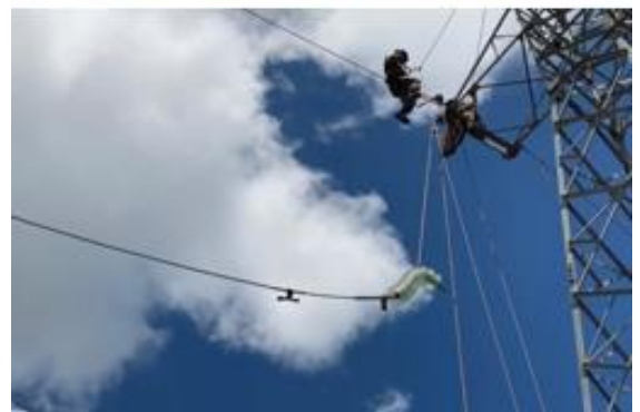
Installation of deadend clamp on the ground
