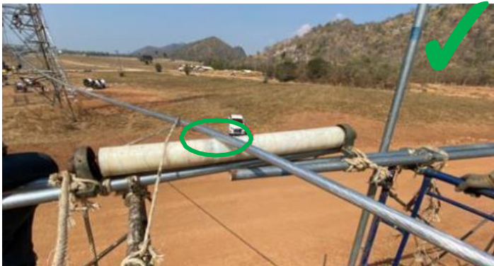
Roller should be used when pulling the conductor over obstacles
