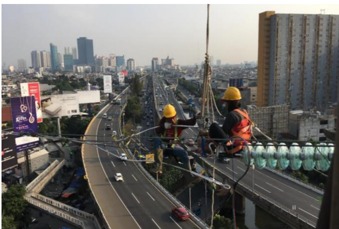
Installation of Deadend clamp on the tower
