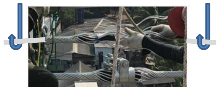
Installation of Armor rod and suspension clamp
