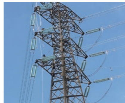
Installed ACFR (Twin Bundle)
