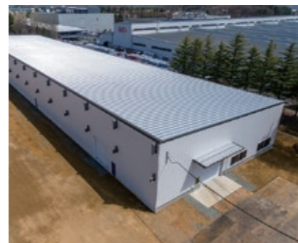
Kitakami CFCC Plant
