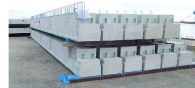
Photo-3 Finished PC Hollow Girders
