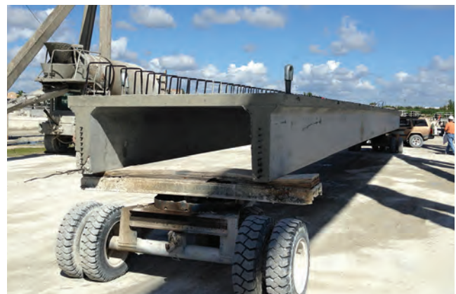
Completion of double-tee beam for the Innovation Bridge in Florida.
