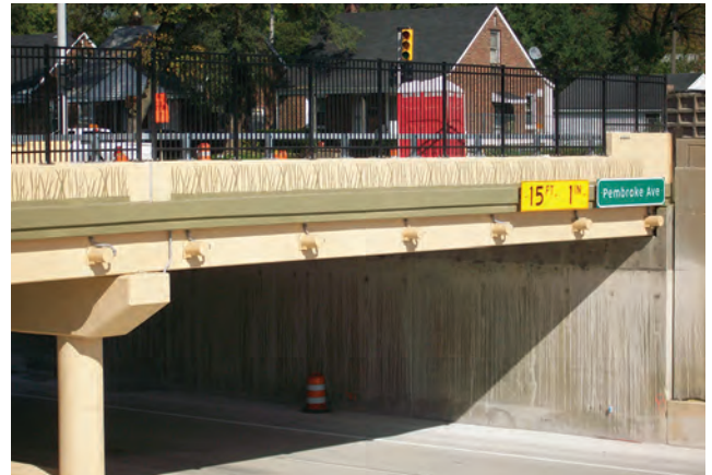
Completion of the Pembroke bridge over Southfield Freeway in Michigan.
