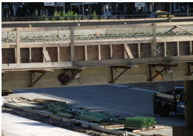
End of transverse posttensioning strand for the Pembroke bridge in Michigan.
