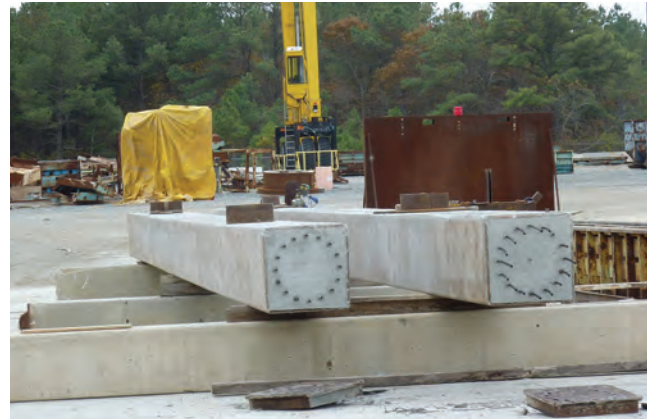
Completed precast concrete piles for the Nimmo Parkway bridge in Virginia.
