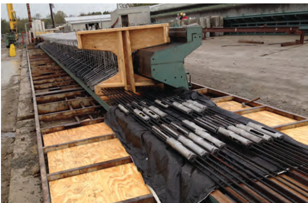
Fabrication of the beam for the KY 70 bridge in Kentucky.
