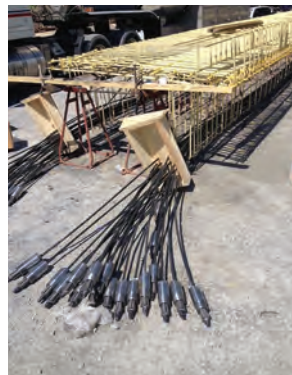
Installation of anchoring devices for the Kittery overpass bridge in Maine.
