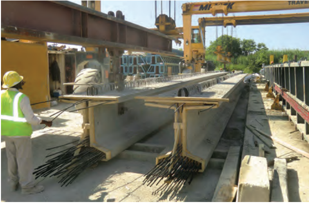
Removing beams from forms for the Route 49 bridge in Virginia.
