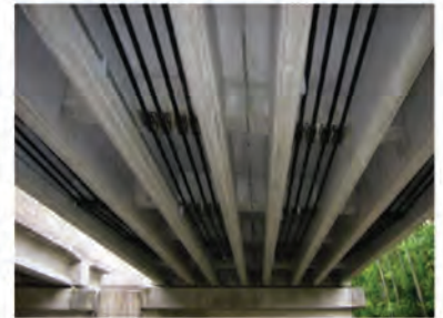
CFCC 1X37 \phi 40.0mm (1.6in) (Post-tensioning)
