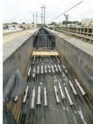
CFCC 1X7 \phi 15.2mm (0.6in) (Pre-tensioning)
