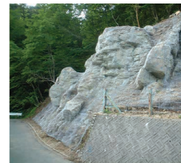
Mighty Net basic elements, high-strength thick net and flexible wire rope, follow the terrain features and stabilize slopes with uneven surfaces.
