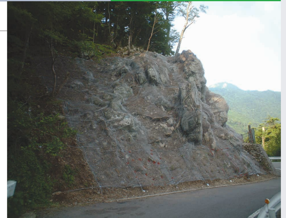
Mighty Net basic elements, high-strength thick net and flexible wire rope, follow the terrain features and stabilize slopes with uneven surfaces.
