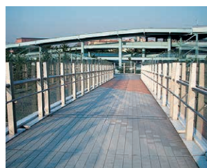
Fence to prevent throwing of objects (pedestrian bridge)
