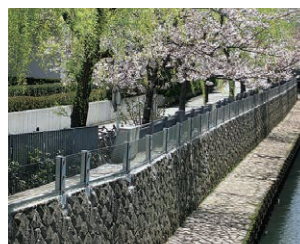
Water cutoff fence
