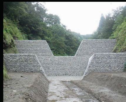
Erosion Control Construction
