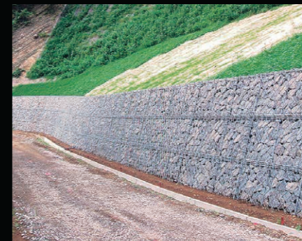
Mountainside soil-retaining construction / Retaining wall
