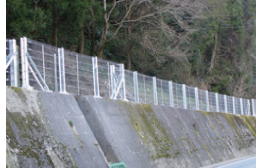
Construction on existing retaining walls
