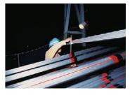
After erection of deck, wires are wrapped on main cable for corrosion protection.
